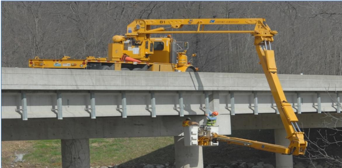
A condition rating is assigned for the bridge’s deck, superstructure and substructure. The lowest rating of the three components is considered the bridge rating. This also applies to culvert condition rating – item 62.
