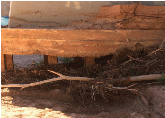
Figure 11 — Scour at a Bridge Pier
