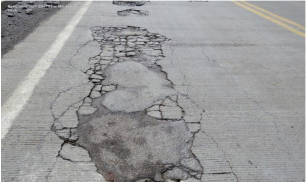
Figure 10 — Cracking and Spalling on a Bridge Deck
