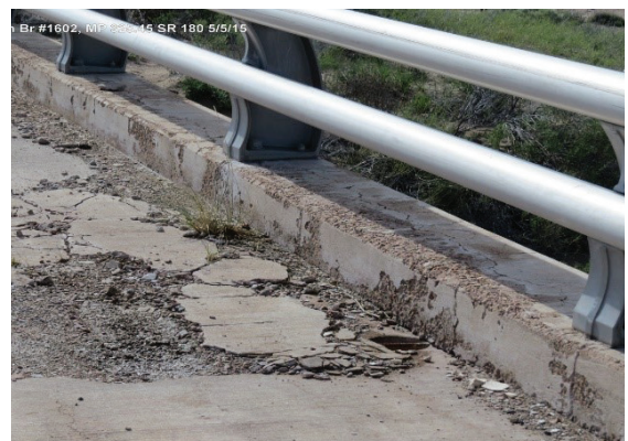
Figure 12 — Scaling on a Bridge Deck
