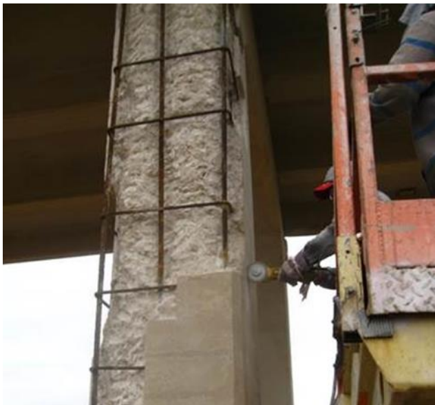
Figure 36. Typical Concrete Substructure Repair Project to Remediate Severe Column Spalling.
