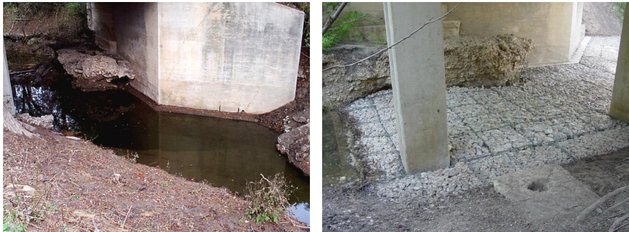
Figure 25. Erosion Repair and Scour Protection (Gabion Mattresses).
