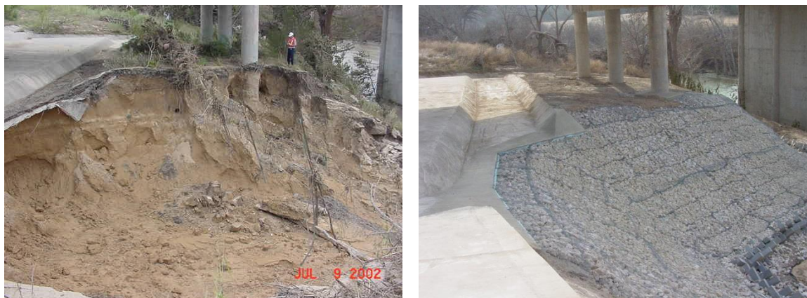
Figure 26. FM 474 @ Guadalupe River in the San Antonio District—Erosion Repairs and Installation of Embankment Protection Measures (Gabion Mattresses).
