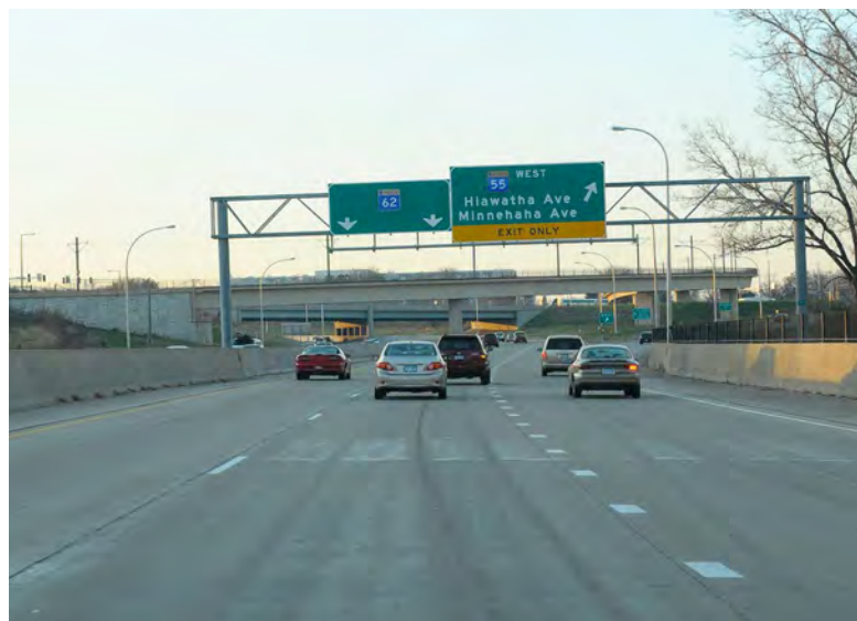
Figure 6-17: Overhead Sign Structure
